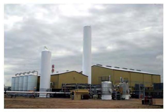
NOVA Chemicals produces hydrogen as a co-product of ethylene manufacturing at our facilities in Joffre, Alberta. We are preventing the creation of additional greenhouse gas emissions (associated with hydrogen production for industrial use) by making this co-product available commercially after processing at our Hydrogen Off-Gas Plant.
